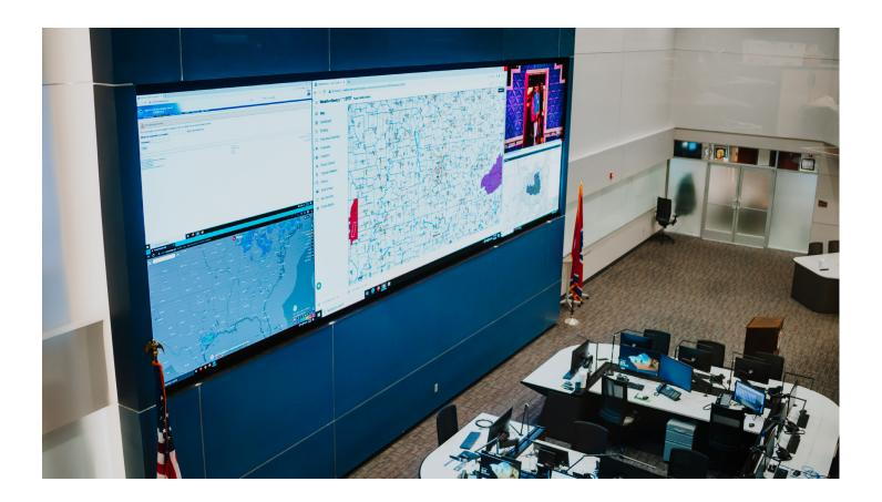
The EOC was previously served by a video wall that was reaching end of life, leading Williamson County EMA to upgrade to the latest display technology with a fine pitch LED video wall from Planar. Installed by audio visual designer and integrator M3 Technology Group, the installation is a nearly 32-foot-wide, 9-foot-high (16x8) Planar® TVF Series LED video wall with a 1.5 pixel pitch (TVF1.5).
