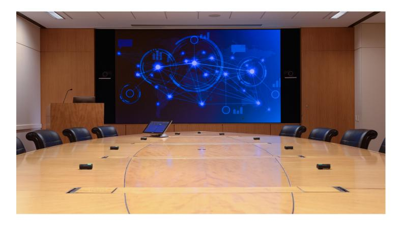
Michetti and his team created an audio visual design featuring LED display technology from Planar--specifically the Planar® TWS Series LED video wall. The proposal included three different pixel pitch options: 1.5mm, 1.2mm and 0.9mm.
