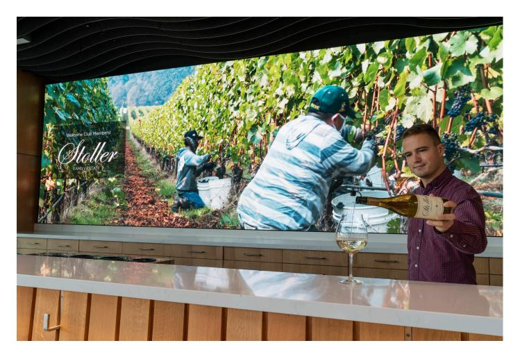
Installed by technology integrator Diversified, the installation is a 21-foot-wide, 6.5-foot-tall Planar® CarbonLight™ CLI Series LED video wall in a 13x4 configuration with a 1.9mm pixel pitch (CLI1.9).
